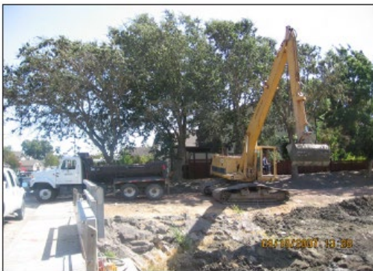
Figure 7. Example of a long-reach excavator that will be used from the north to remove sediment and Ludwigia from Laguna 1 and Laguna 2
